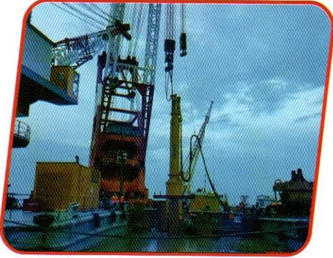
PDA Test at TD4A (after Static Load Test)
