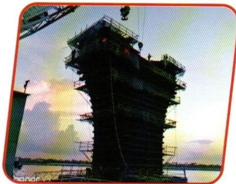
Pile Cap, Pier Shaft & Pier Cap
