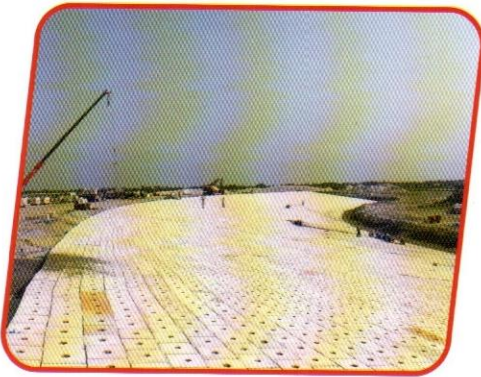
River Training Works Activities
