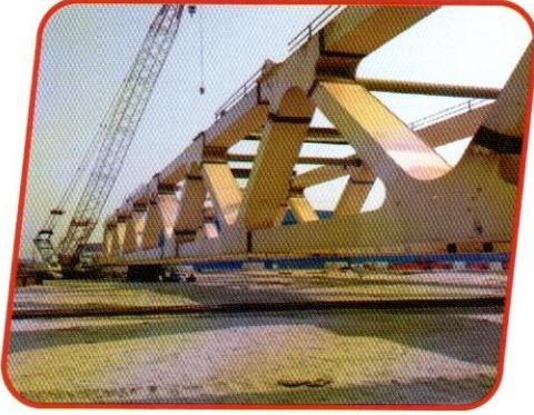
Truss Assembling
