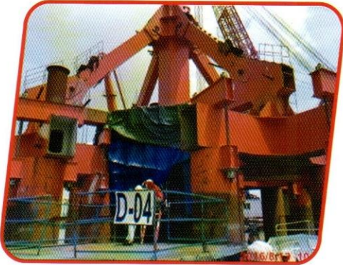
Static load test of TD4A stage-1
